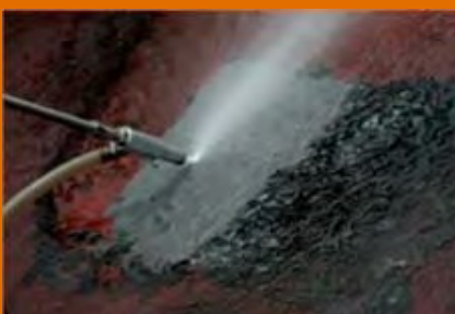
Surface sand blasting
