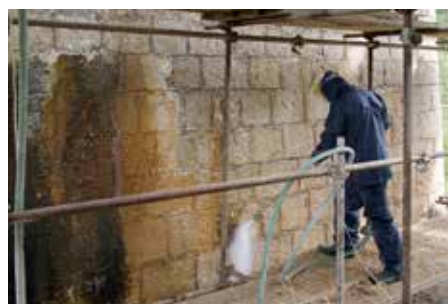
Cleaning building scaffolding
